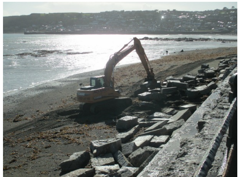
Repairs to Penzance promenade get under way
