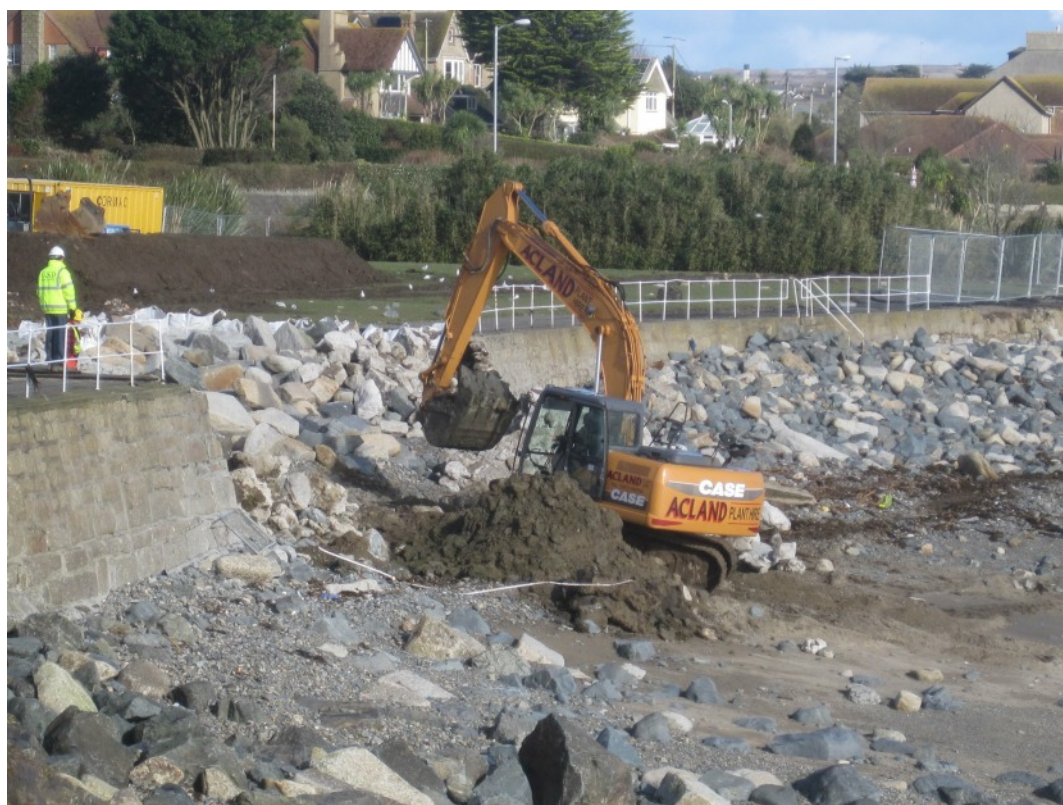
A start on repairs at Newlyn Green
